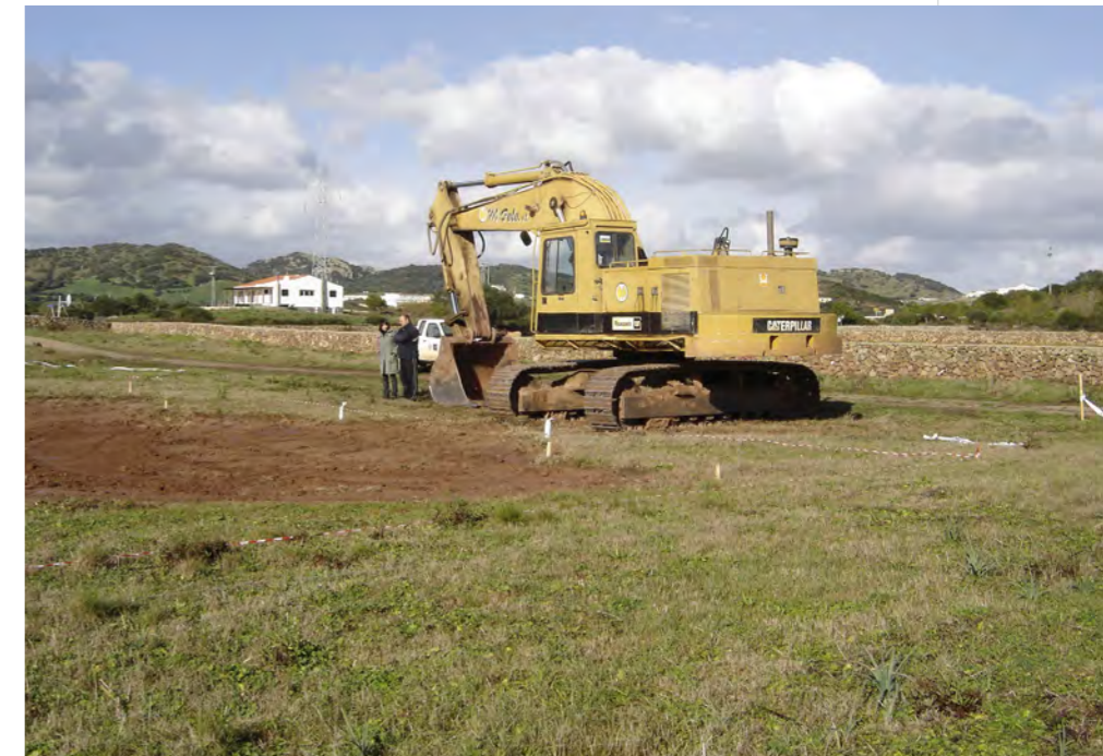
Excavation of an experimental temporary pond for educational purposes in Santa Eularieta
